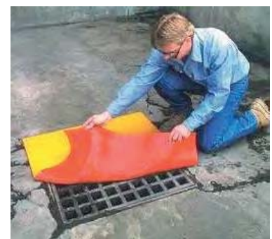
Figure 12 - temporarily isolating a drain with an impervious mat
