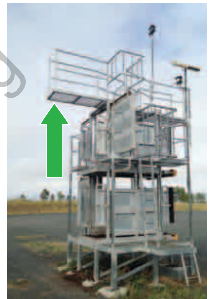
FIGURE 14c Cross loading structure with walkway enabling safe access to the top of the crate and from one crate to another
