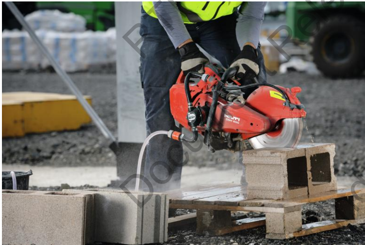
Figure 2: on tool water suppression (source: Hilti Australia)
