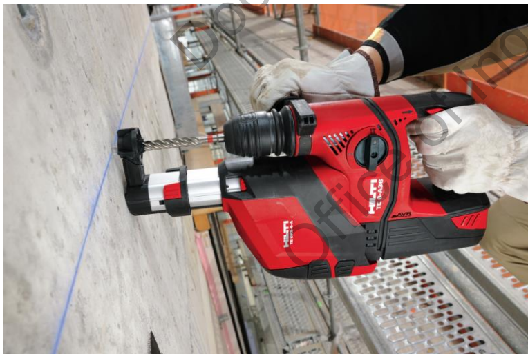
Figure 6: on tool dust extraction (Source: Hilti Australia)
