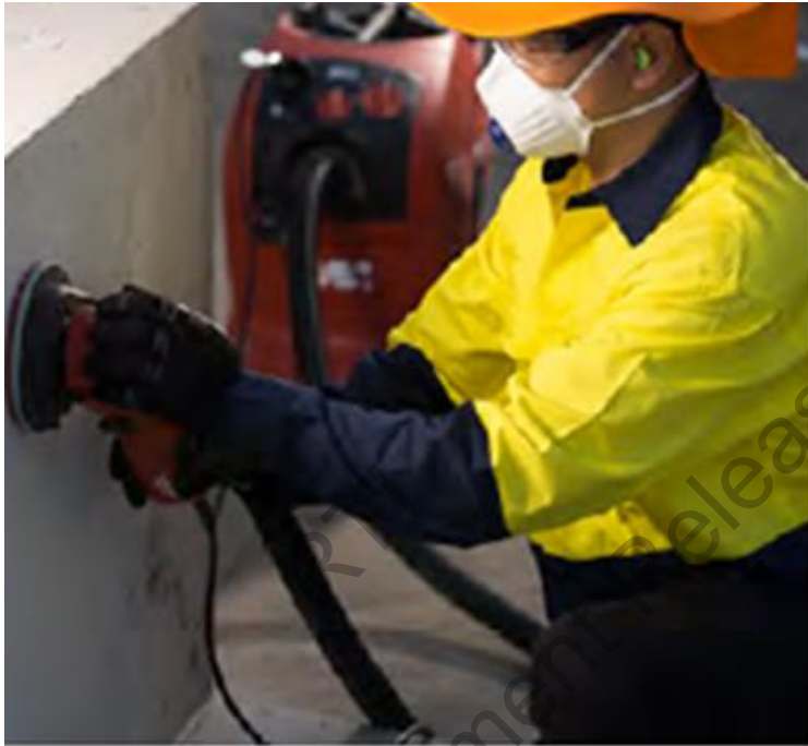
Figure 5: On tool dust extraction (Source: WorkSafe Queensland)
